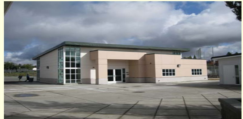
Windsor Middle School Music Building
