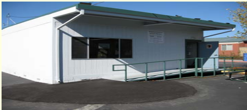
Windsor Oaks Academy Growth Project
